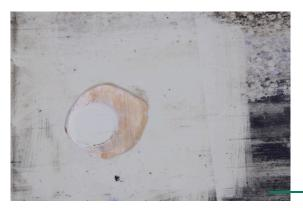
**5.** Area around damage, ready to repair
