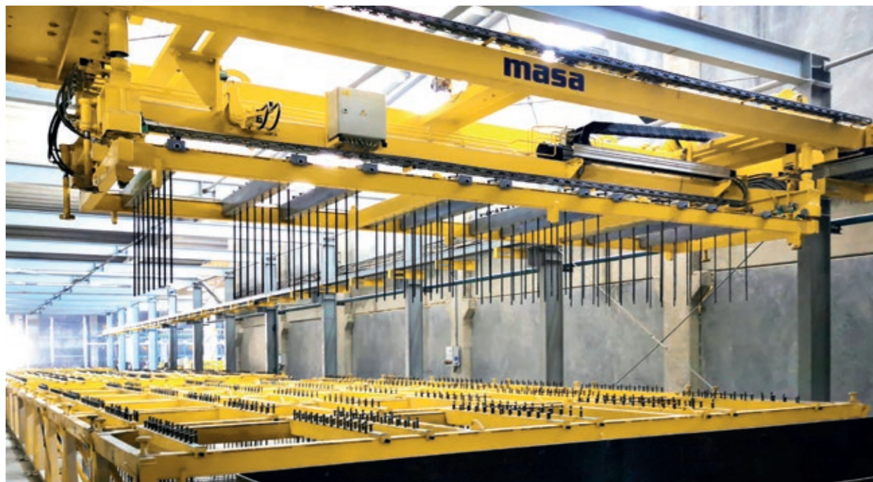
Preparation of reinforcement
